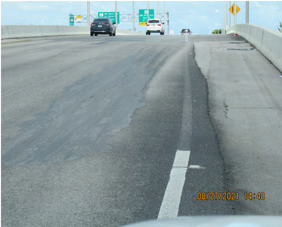
DETERIORATED WHITE EDGELINE STRIPING
