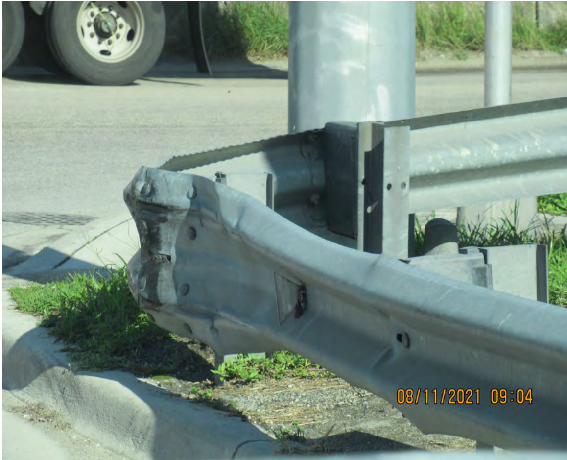
DAMAGED GUARDRAIL
