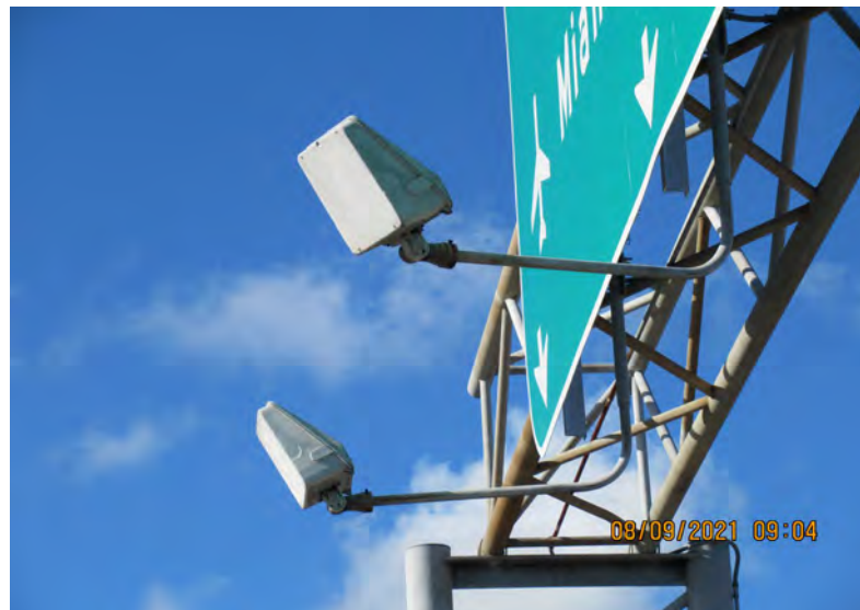
TWISTED LUMINAIRE (STRUCTURE # 87S422)
