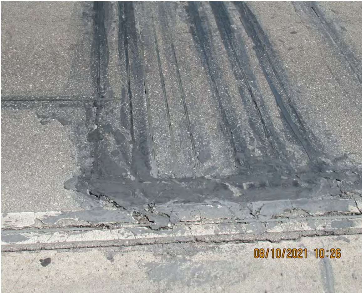
DETERIORATED TOLLS LOOP DETECTOR SEALANT
