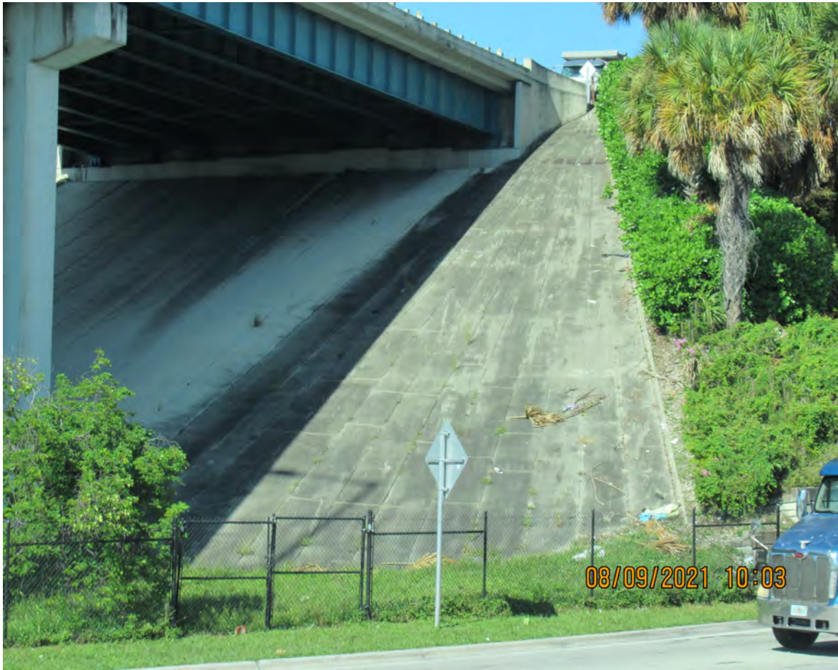
DETERIORATED CLASS V COATING ON SLOPE (BRIDGE # 870238) (TYPICAL THROUGHOUT THE CORRIDOR)
