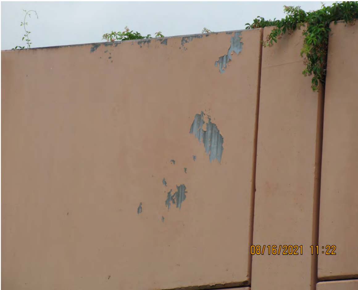
DETERIORATED CLASS V COATING ON SOUND WALLS (TYPICAL THROUGHOUT THE CORRIDOR)
