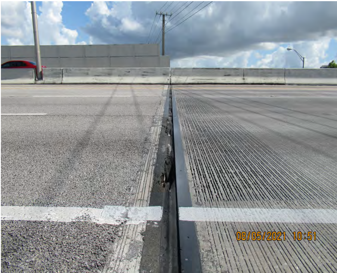
DETERIORATED EXPANSION JOINT (BRIDGE # 870708)
