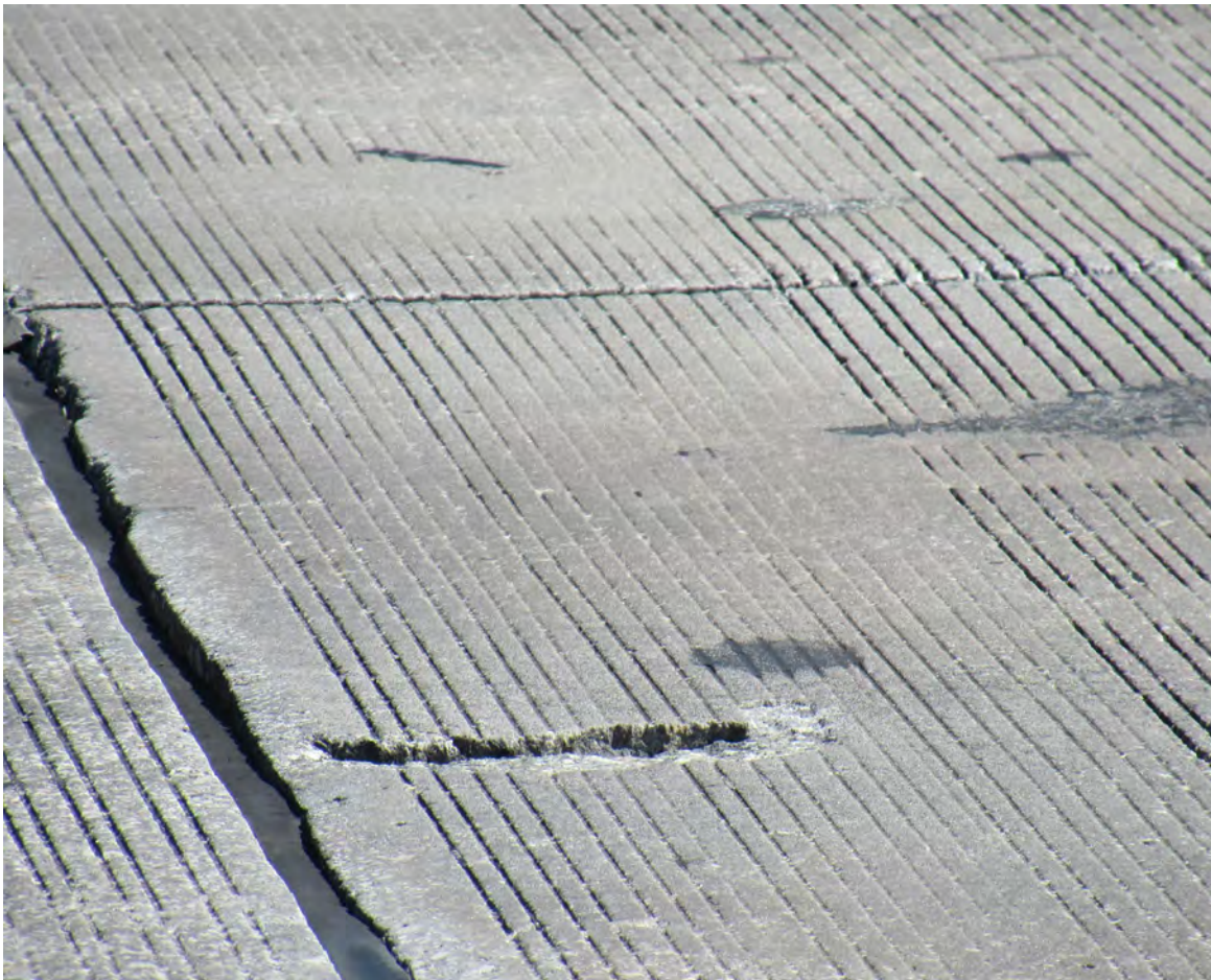
SPALLS ON APPROACH SLAB (BRIDGE # 870721)
