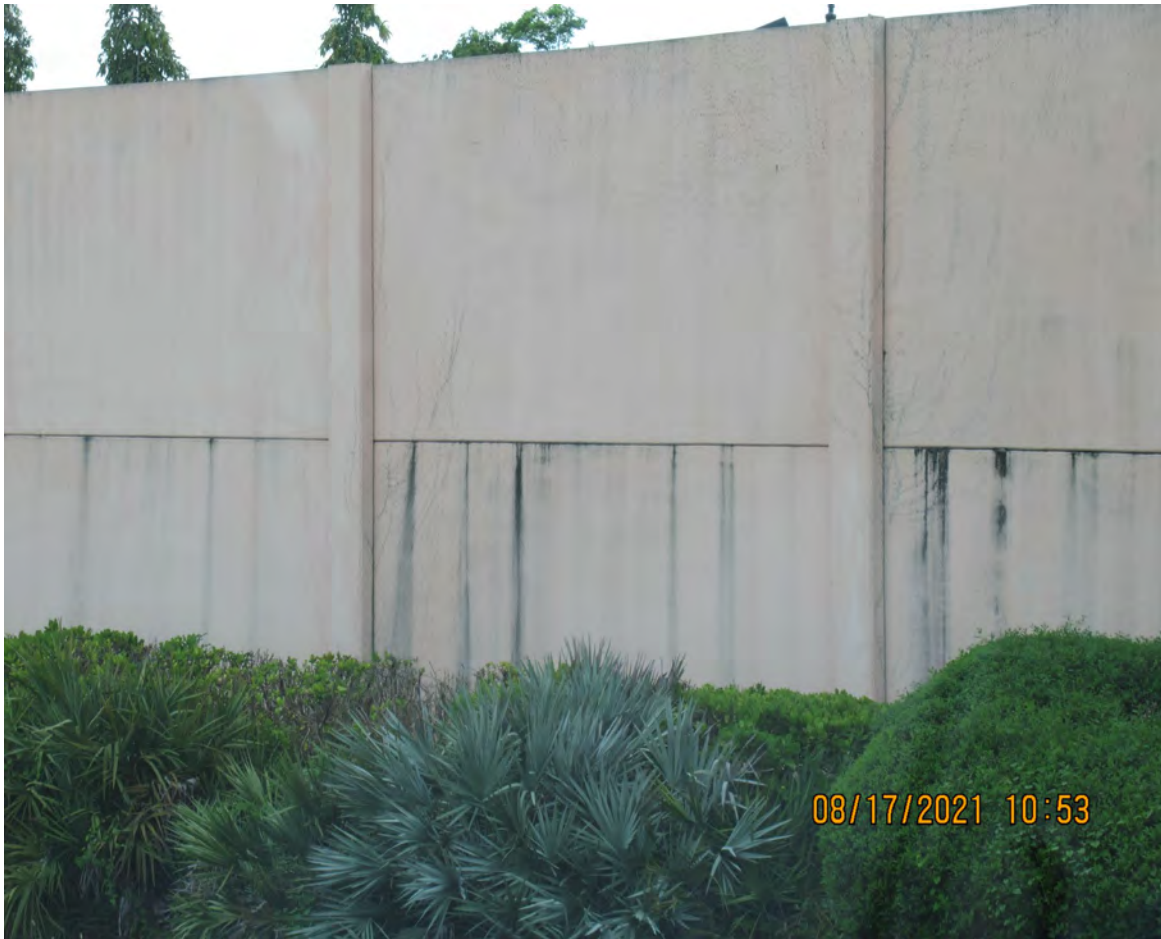
DETERIORATED CLASS V COATING ON SOUND WALL (TYPICAL THROUGHOUT THE CORRIDOR)
