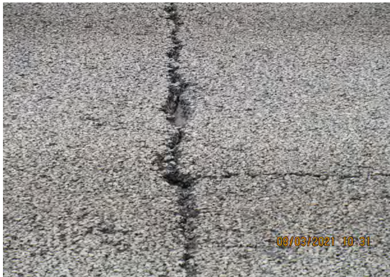
TRANSVERSE PAVEMENT CRACK AT APPROACH SLAB (BRIDGE # 870738)
