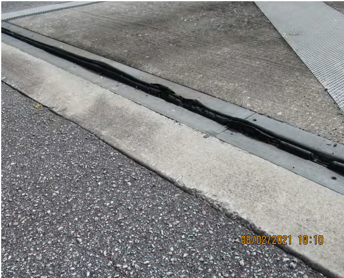
DETERIORATED EXPANSION JOINTS (BRIDGE #870557) TYPICAL THROUGHOUT THE CORRIDOR
