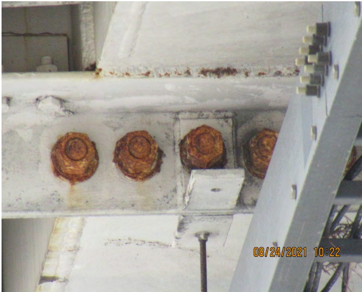
CORROSION ON ORT GANTRY BOLTS (STRUCTURE # 87A253)
