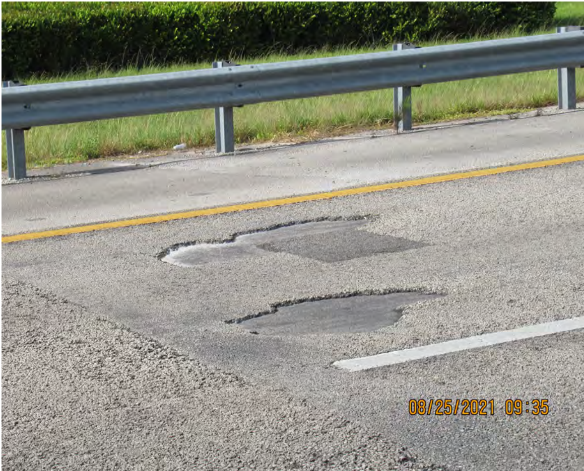
DAMAGED FRICTION COURSE PAVEMENT
