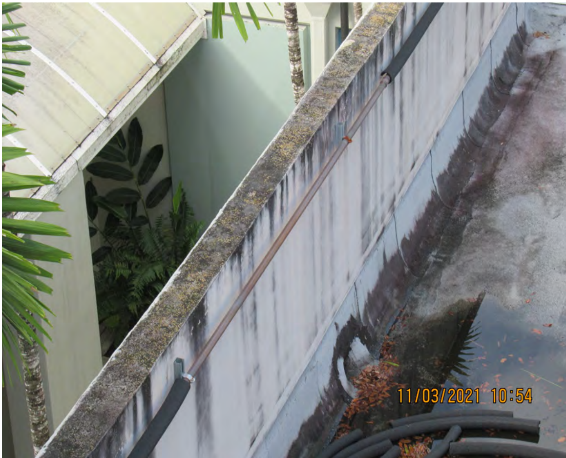
MISSING INSULATION ON REFRIGERANT LINE
