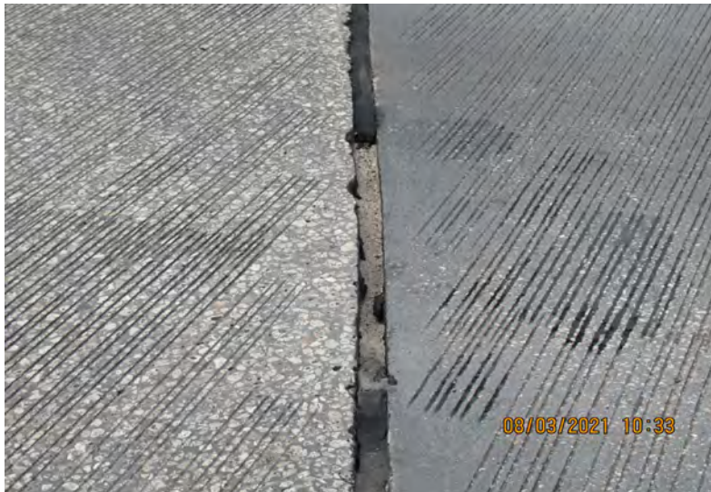
DETERIORATED JOINT SEALANT (BRIDGE # 870738)
