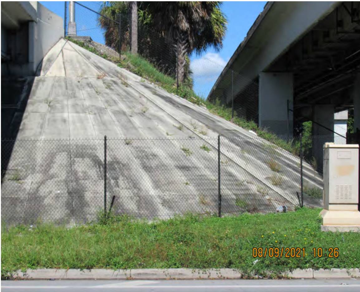
DETERIORATED CLASS V COATING ON SLOPE (TYPICAL THROUGHOUT THE CORRIDOR)
