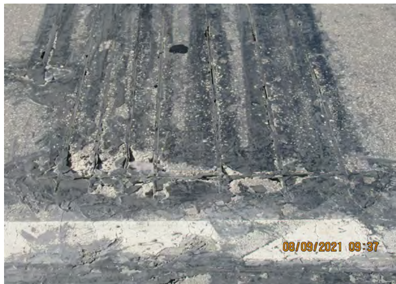
DETERIORATED LOOP DETECTOR SEALANT
