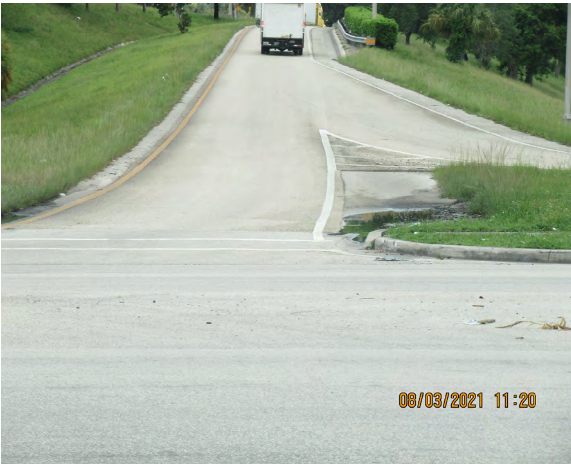
PONDING WATER ON RAMP ENTRANCE
