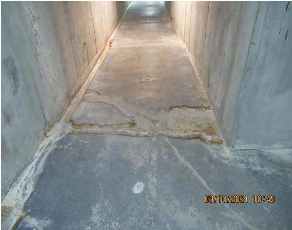
WATER INTRUSION STAINS ON TUNNEL FLOOR
