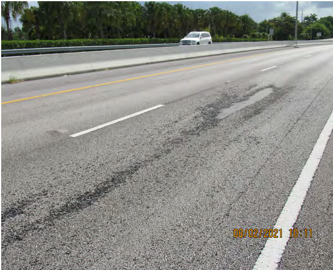
DETERIORATED ASPHALT PAVEMENT
