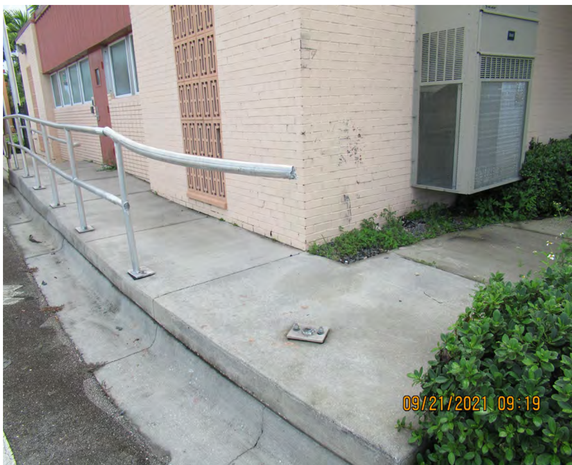
UNREPAIRED DAMAGED PEDESTRIAN RAILING
