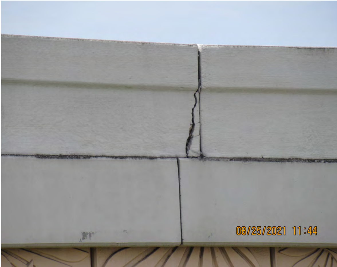
CRACKED BARRIER WALL
