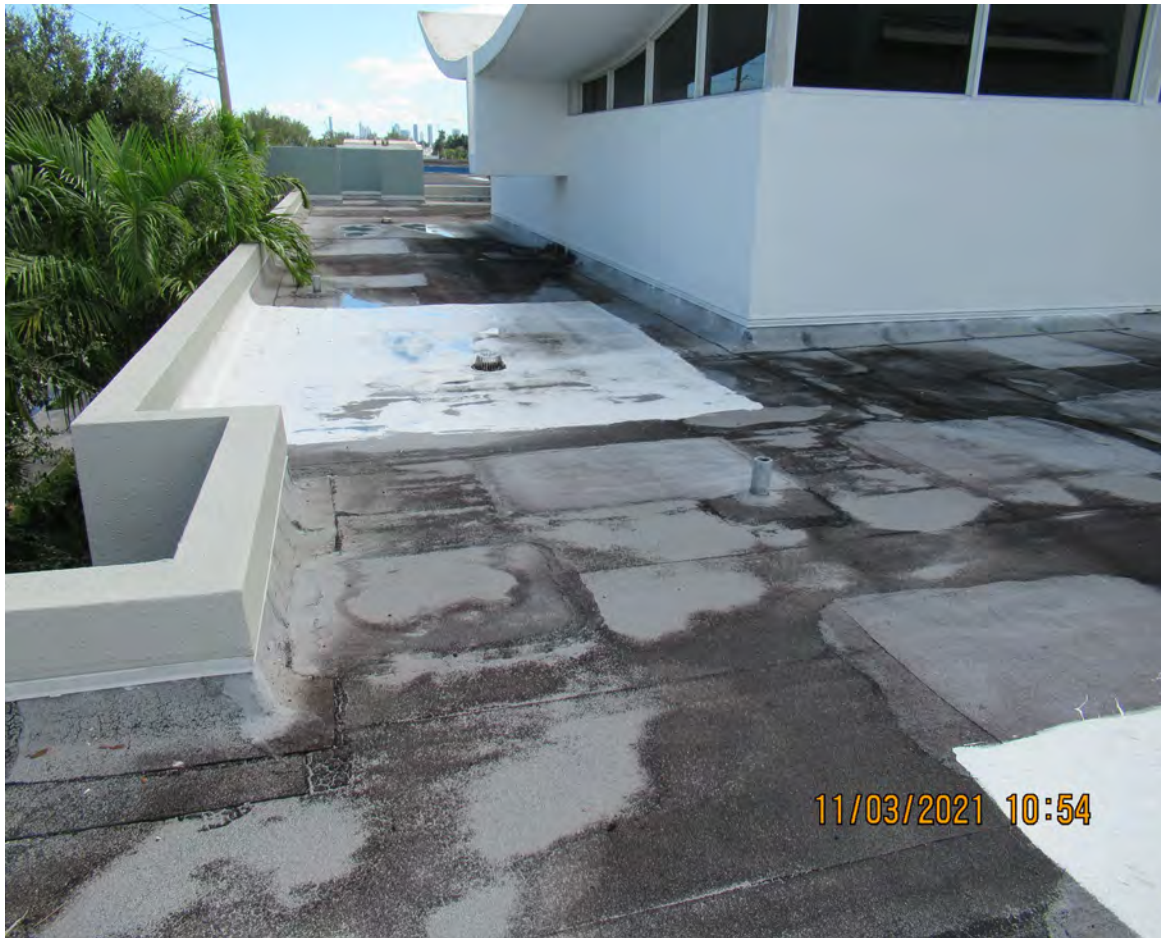
ISOLATED REPAIRS ON ROOF MEMBRANE
