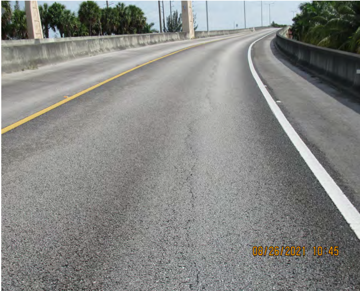
LONGITUDINAL CRACK ON PAVEMENT
