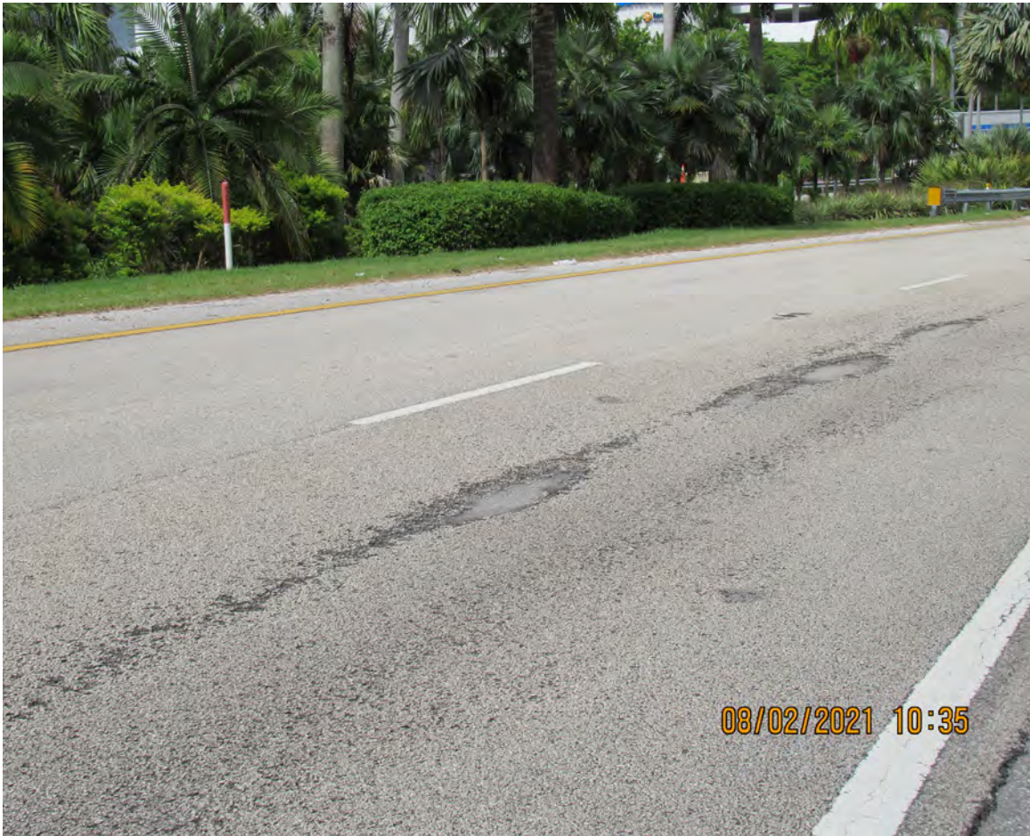
DETERIORATED ASPHALT PAVEMENT
