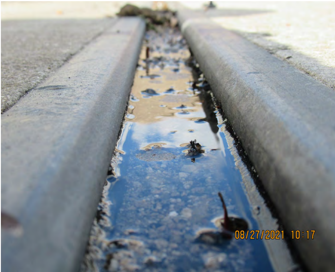
SEDIMENT AND DEBRIS ON BRIDGE EXPANSION JOINTS (BRIDGE # 870966) (TYPICAL THROUGHOUT)
