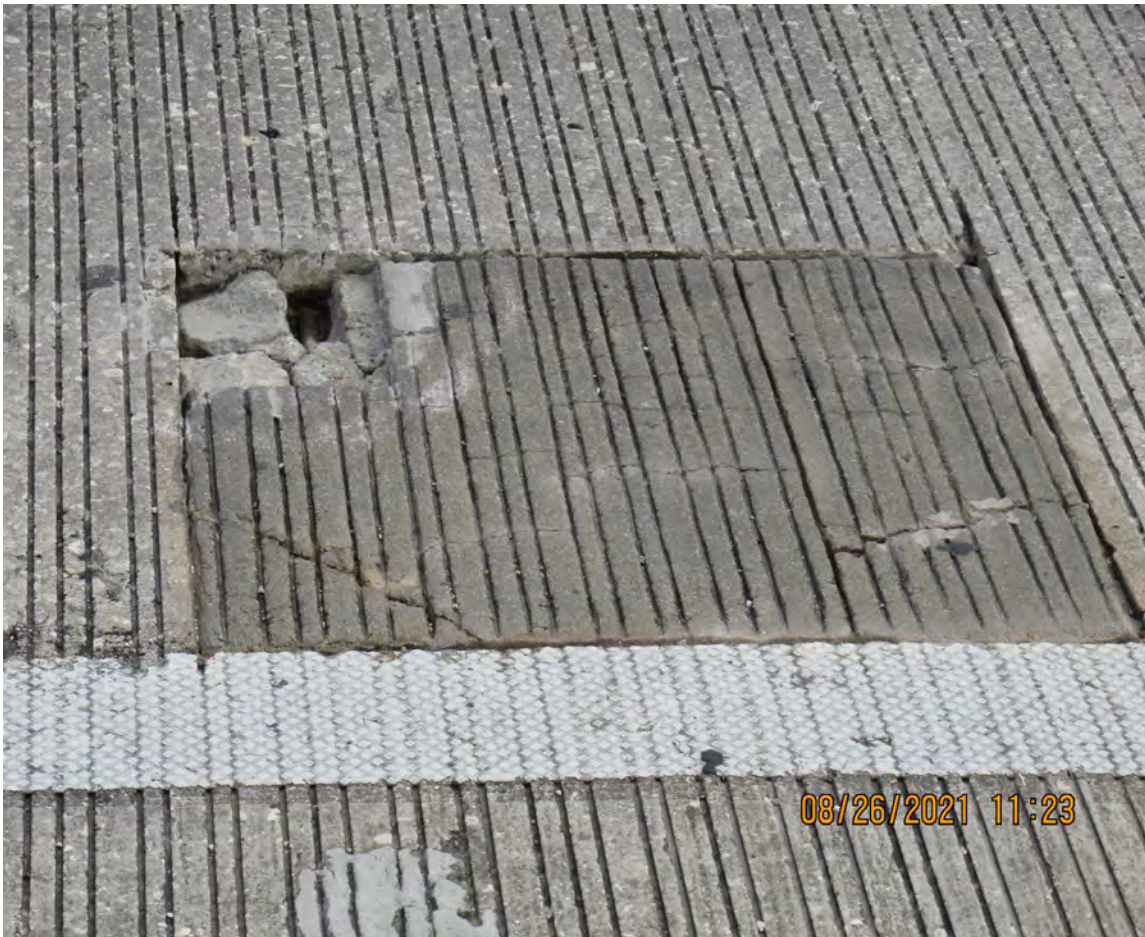
SPALL ON BRIDGE DECK (BRIDGE No. 871002)
