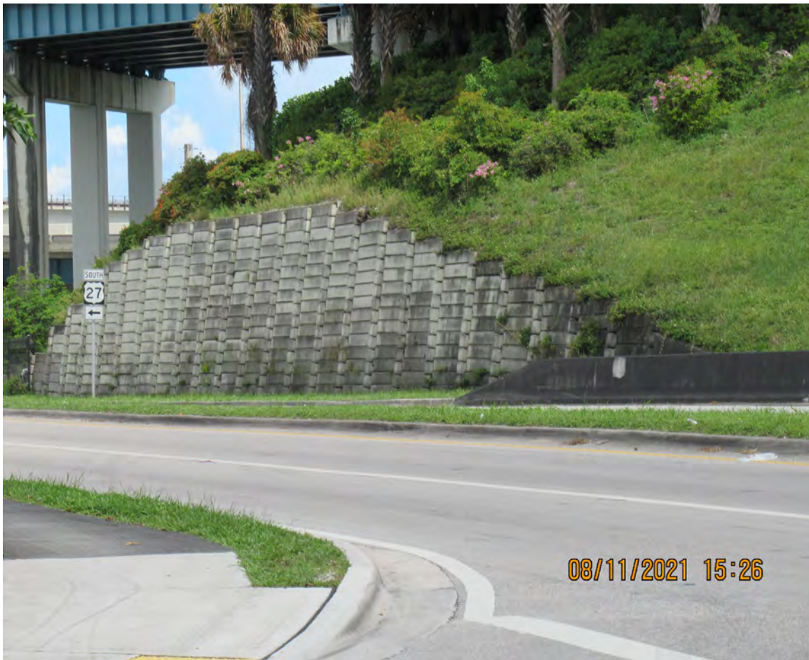
DETERIORATED CLASS V COATING ON RETAINING WALL
