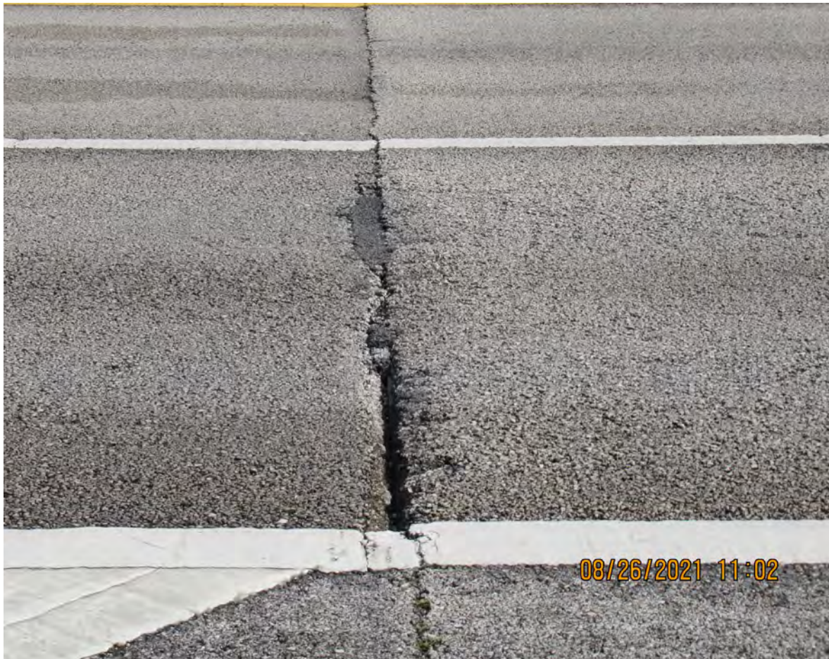
TRANSVERSE CRACK ON PAVEMENT AT APPROACH SLAB (BRIDGE No. 871002)
