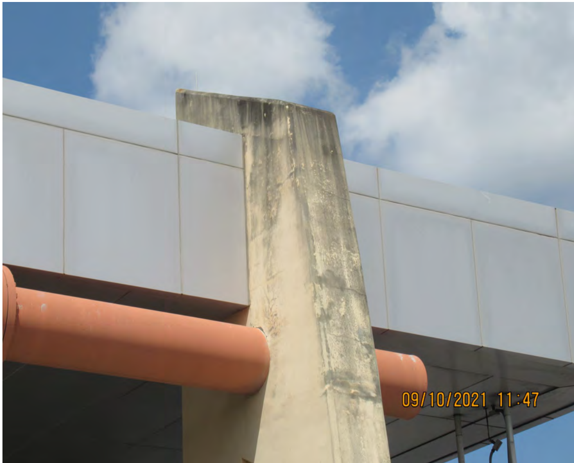
DETERIORATED CLASS 5 COATING ON TOLL CANOPY COLUMNS
