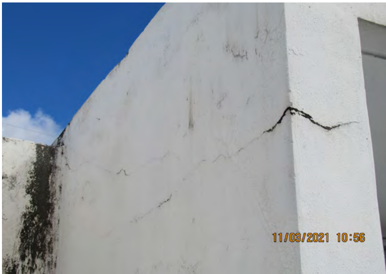
SURFACE CRACKS ON EXTERIOR PARAPET WALL
