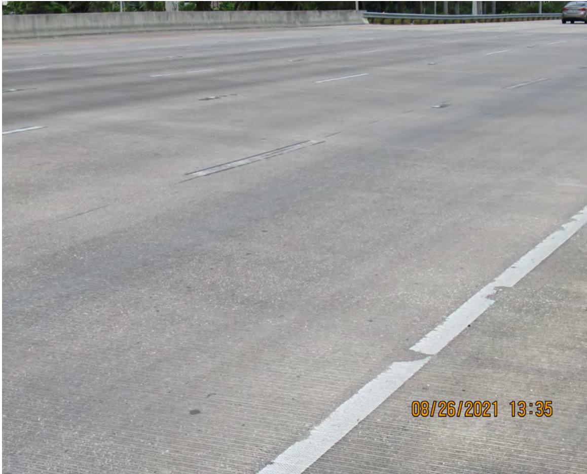
DETERIORATED STRIPING (BRIDGE No. 871010)
