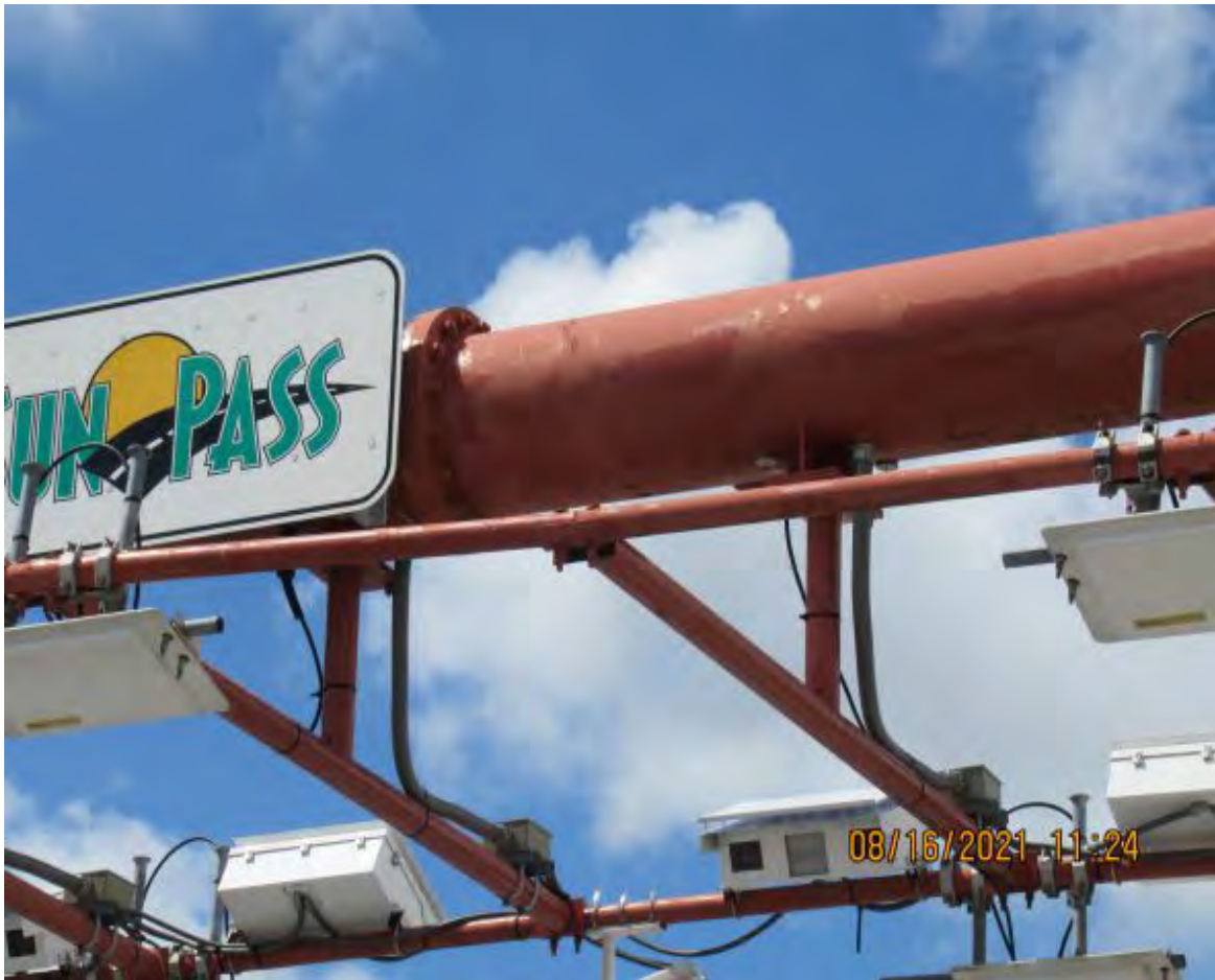
DETERIORATED PAINT ON ORT STRUCTURE UPRIGHTS AND MONOTUBE (STRUCTURE # 87S937)
