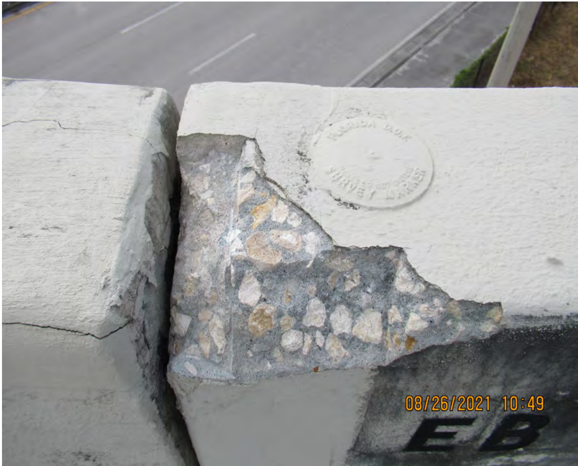
SPALL ON TRAFFIC RAILING (ABUTMENT 1, BRIDGE No. 871008)
