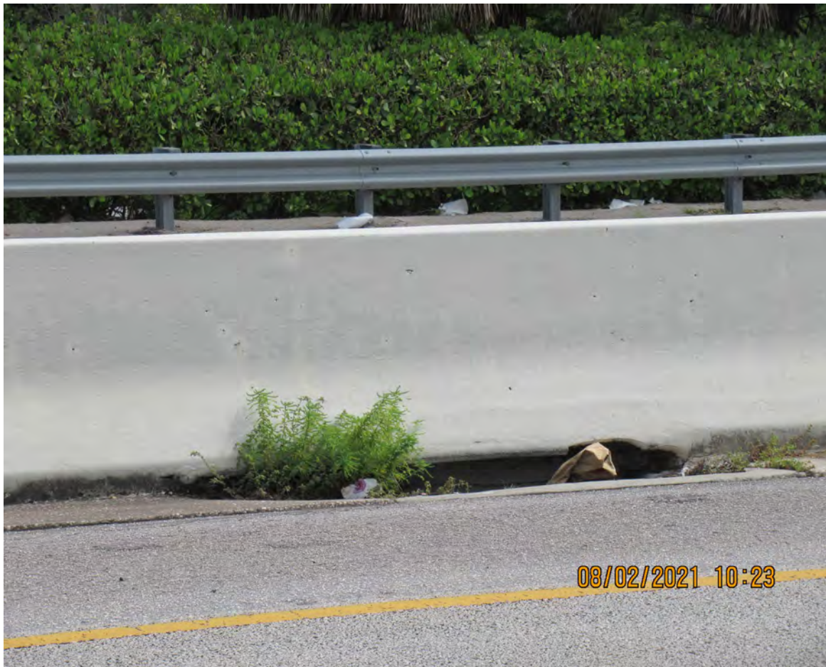
SILTED INLET (TYPICAL THROUGHOUT THE CORRIDOR)
