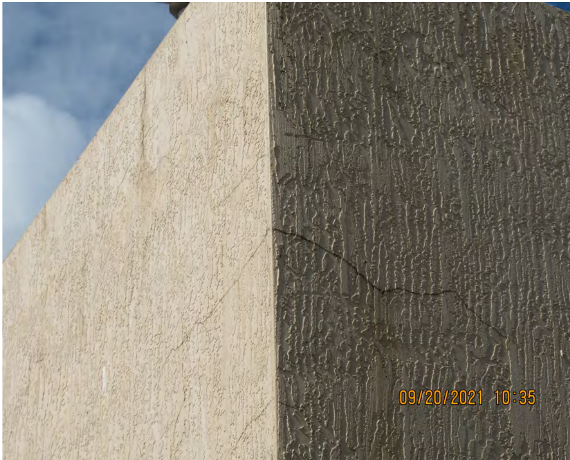
CRACKS ON STUCCO
