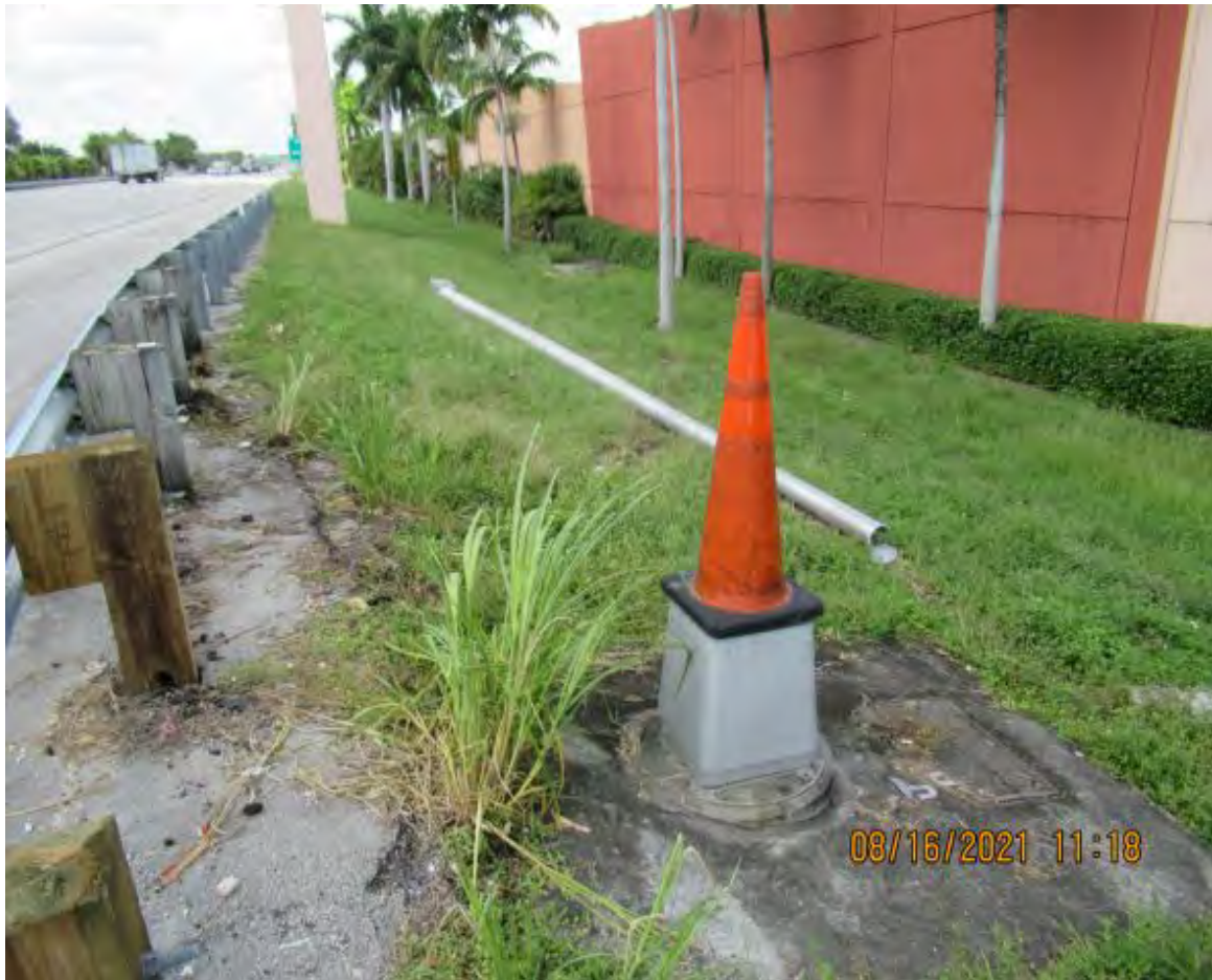
DAMAGED LIGHT POLE DUE TO VEHICULAR ACCIDENT (POLE # 02-74 16)
