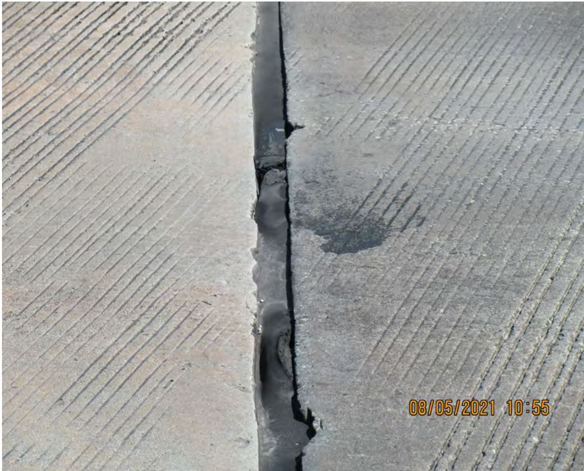
DETERIORATED EXPANSION JOINT SEALANT (BRIDGE # 870720)
