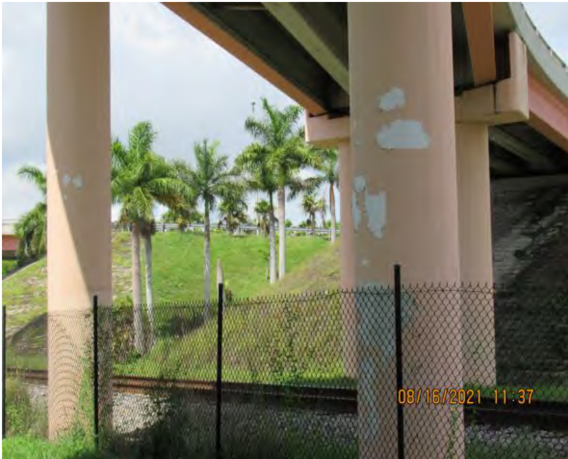
DETERIORATED CLASS V COATING ON BRIDGE COLUMNS (BRIDGE # 870543)
