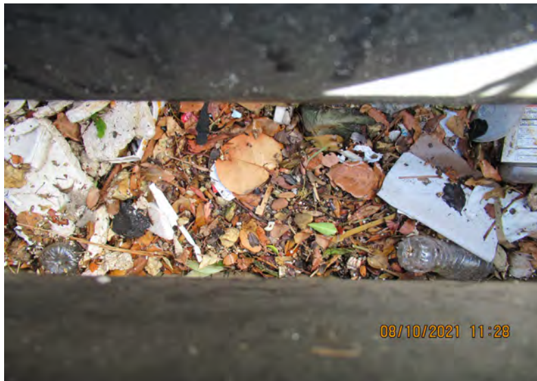
SILTED DRAINAGE INLET (TYPICAL THROUGHOUT THE CORRIDOR)
