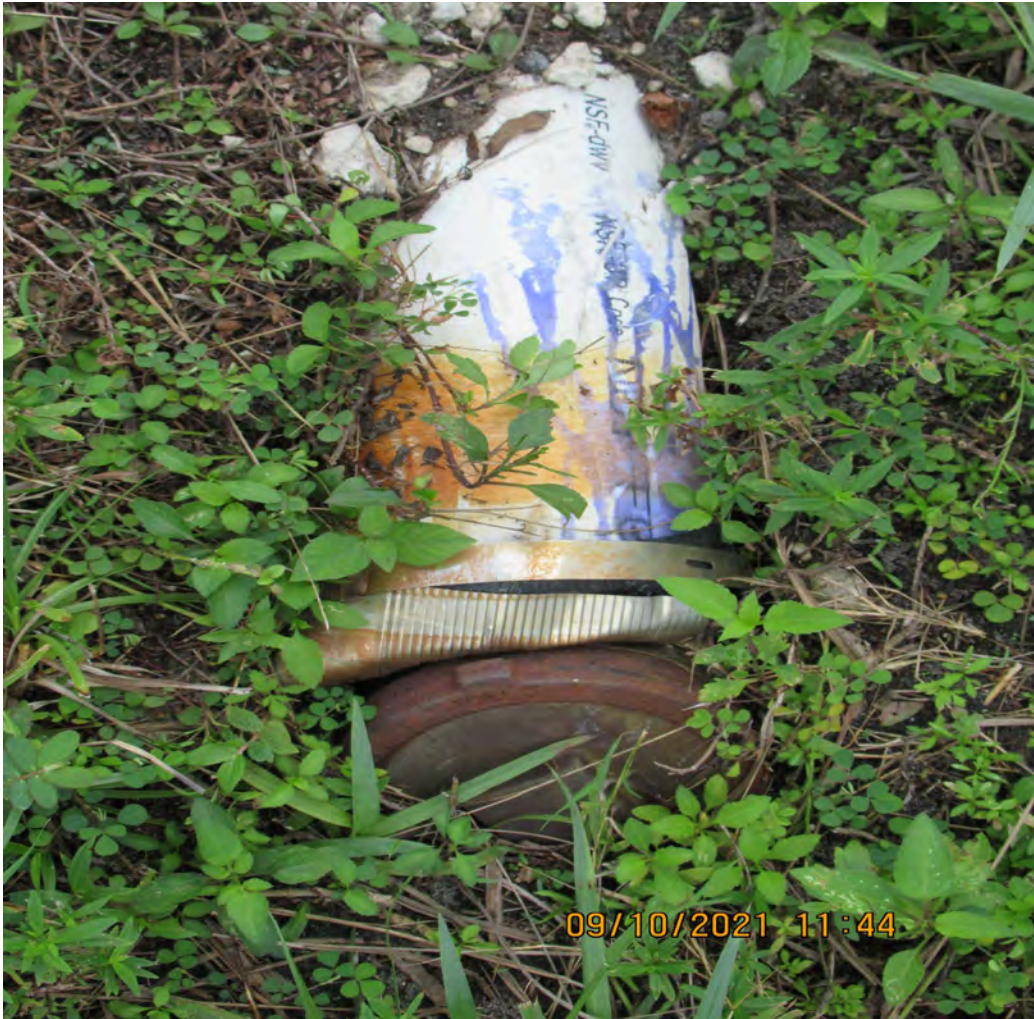
IMPROPER SEWER CLEANOUT INSTALLATION
