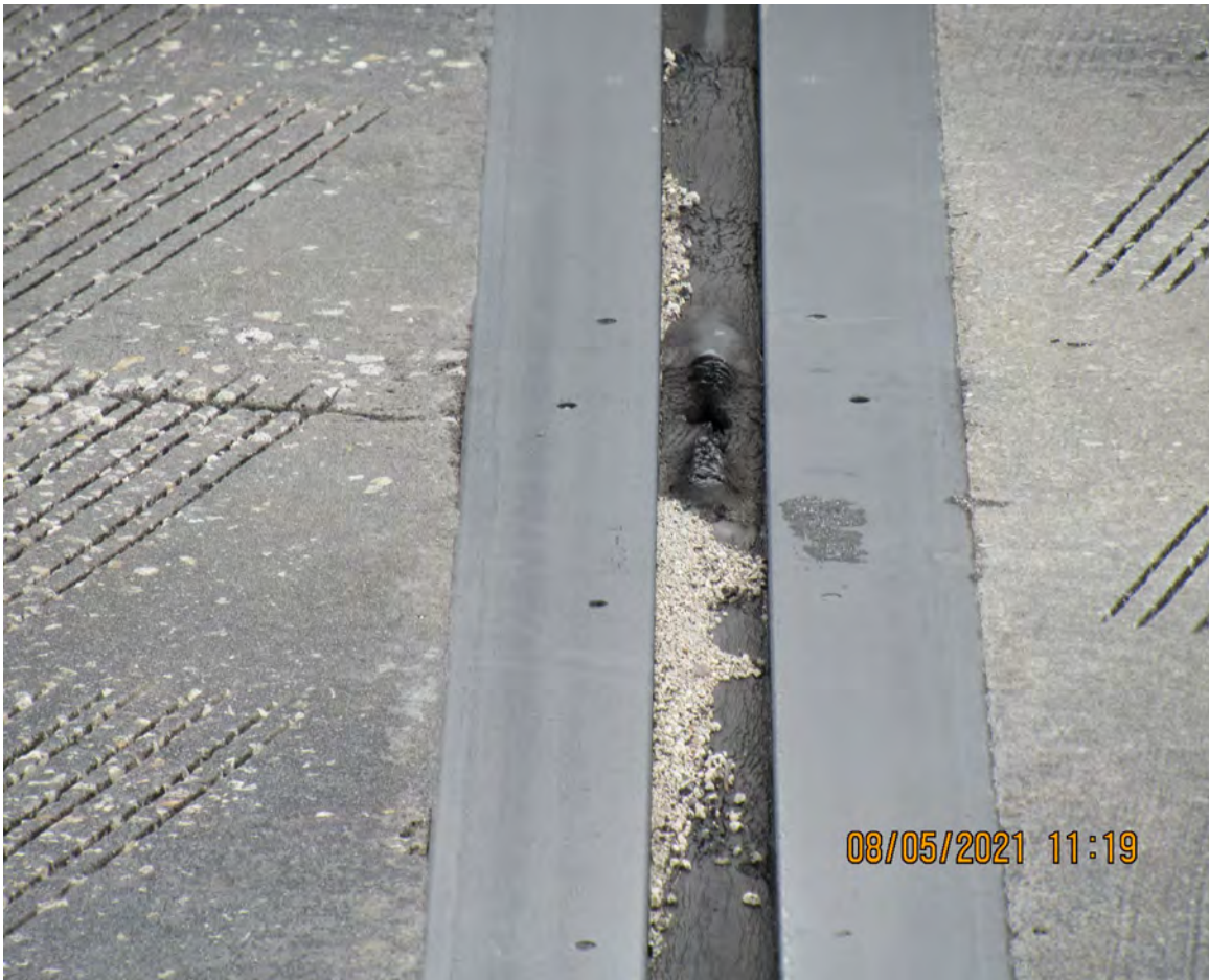
DETERIORATED BRIDGE JOINT (BRIDGE # 870740)
