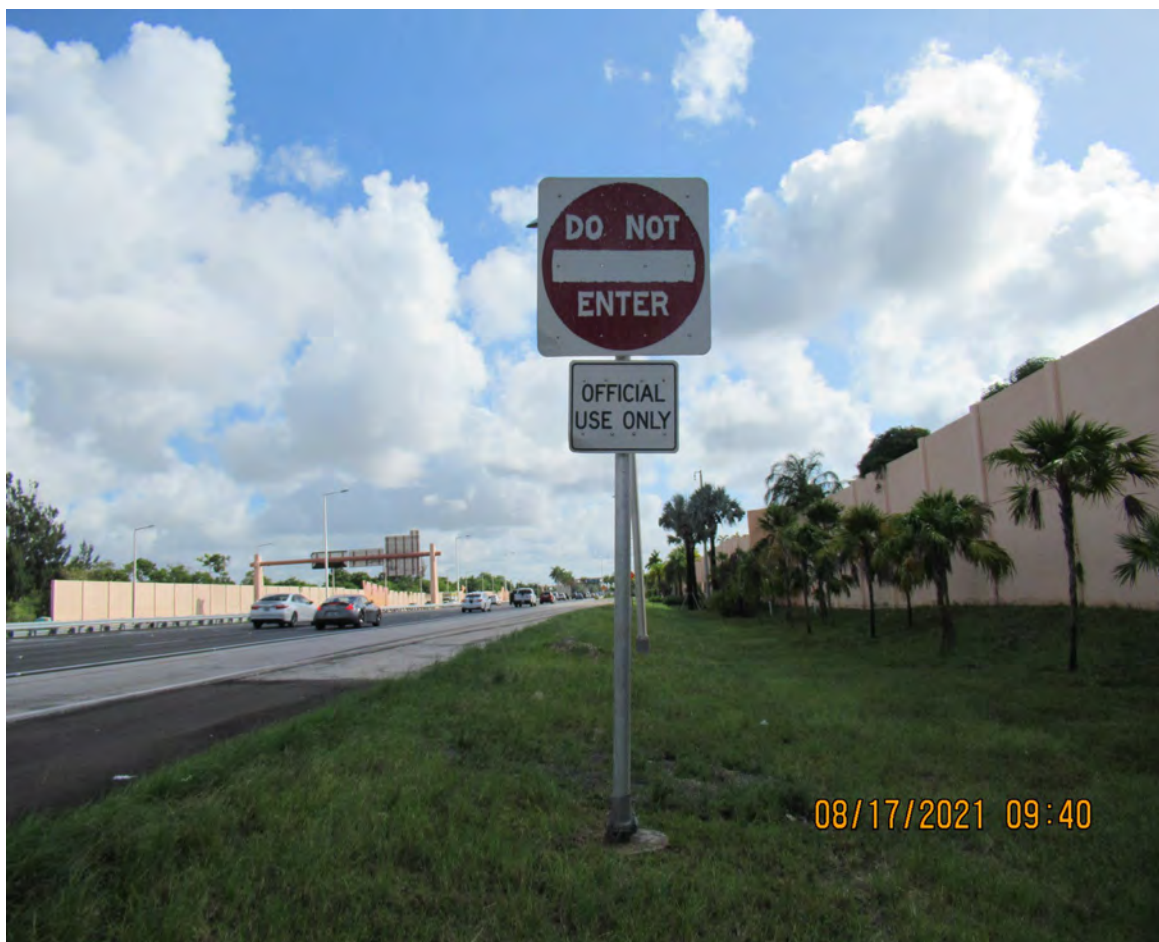
DETERIORATED REFLECTIVE SHEETING ON DO NOT ENTER SIGN (TYPICAL OF TWO SIGNS)
