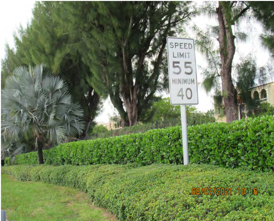
DETERIORATED REFLECTIVE SHEETING ON SPEED LIMIT SIGN
