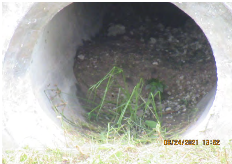
SEDIMENTATION INSIDE CROSS DRAINS
