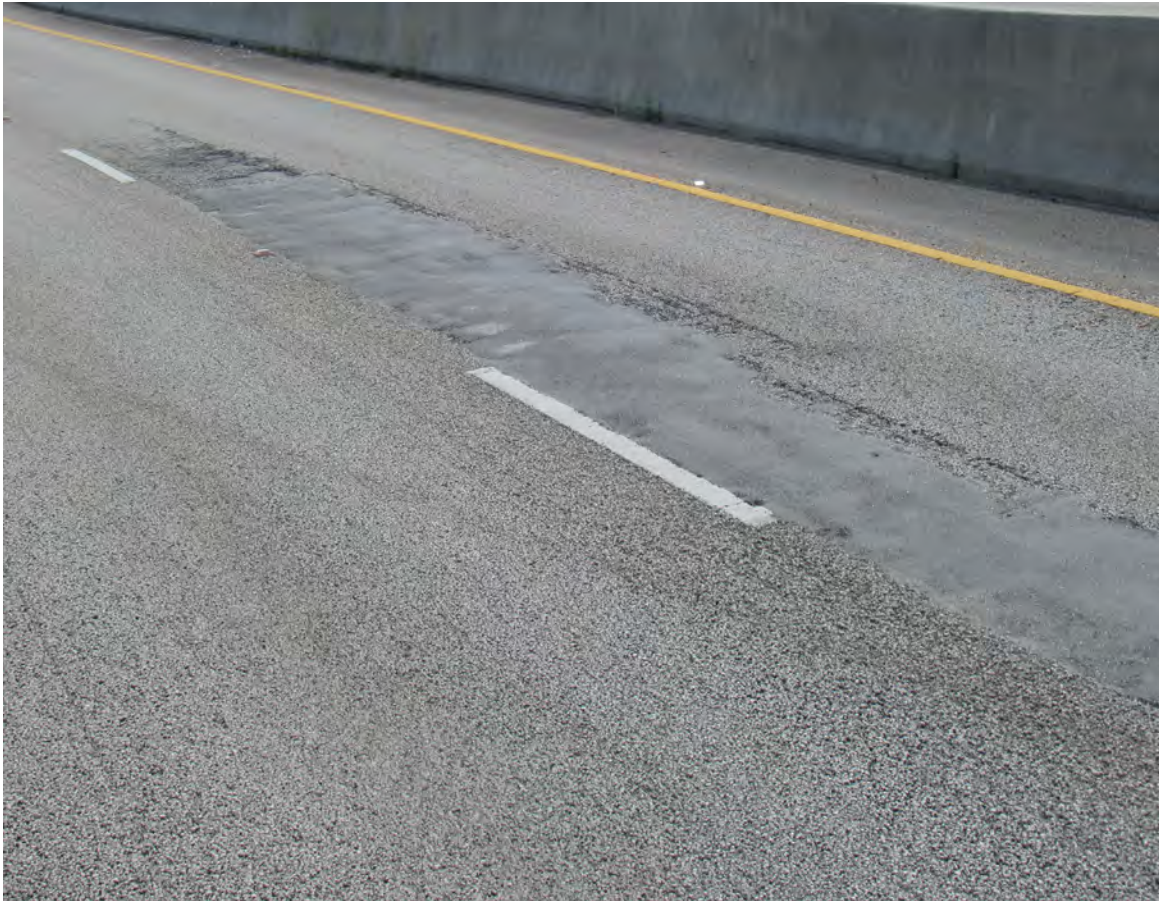
DETERIORATED ASPHALT REPAIR
