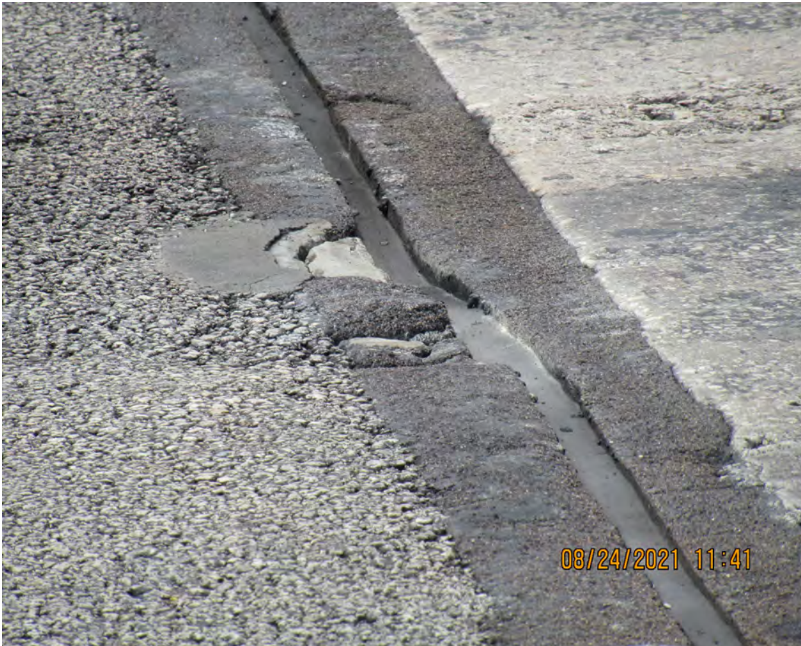
DAMAGED POLYMER NOSING JOINT HEADER (BRIDGE No. 870138)
