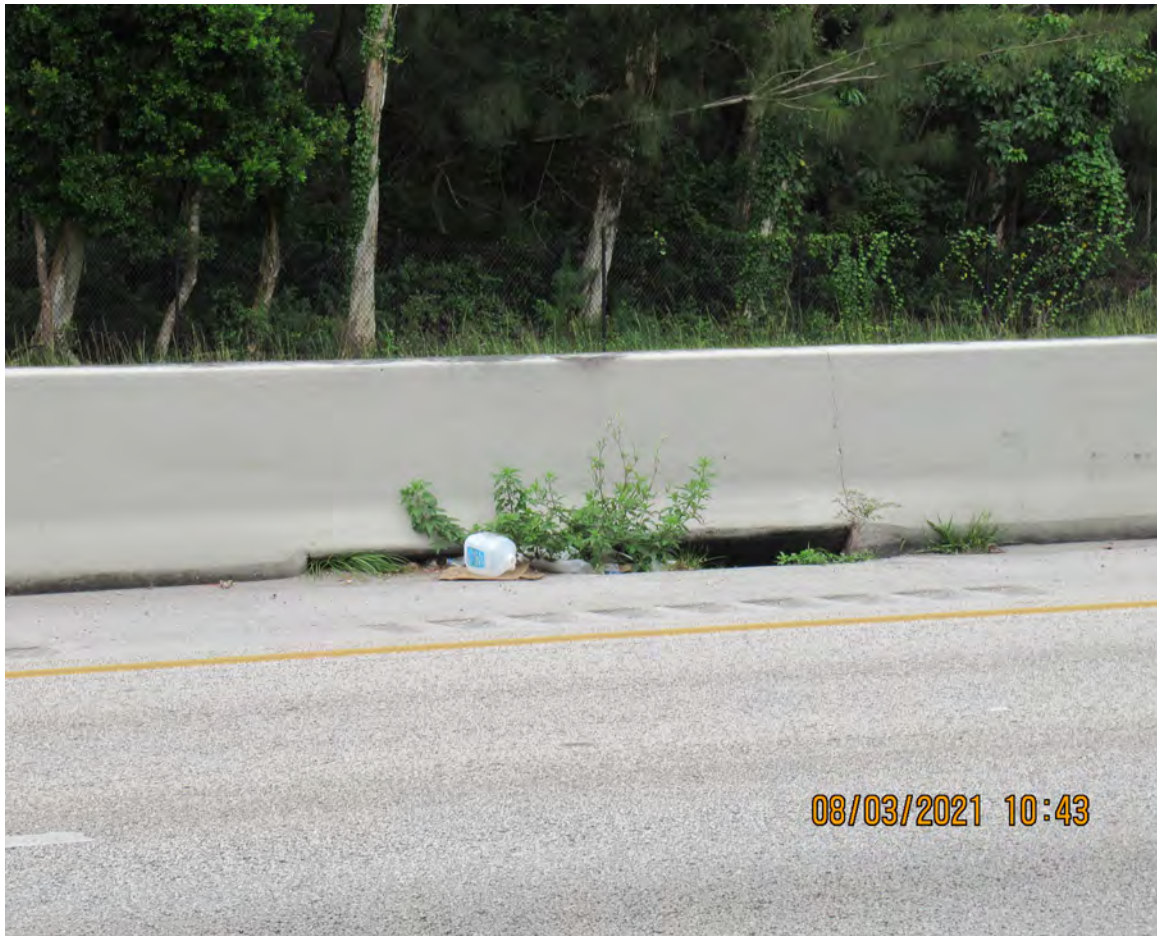
SILTED DRAINAGE STRUCTURE (TYPICAL TROUGHOUT THE CORRIDOR)
