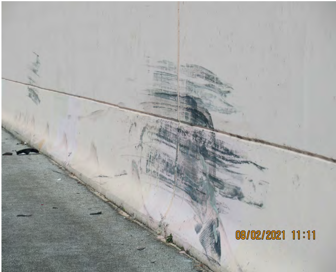
DETERIORATED CLASS V COATING ON BARRIER WALL (TYPICAL THROUGHOUT THE CORRIDOR)
