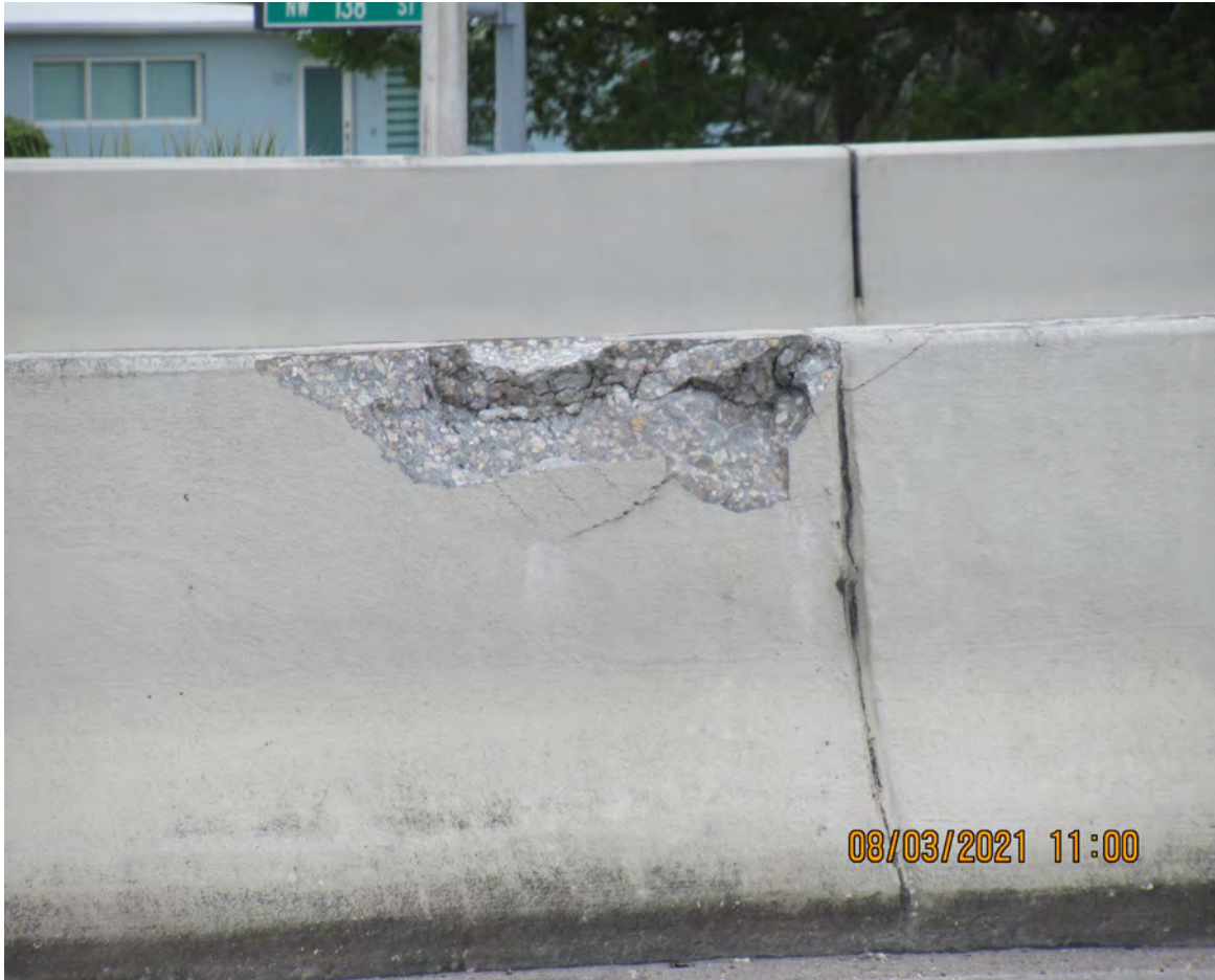
DAMAGED MEDIAN BARRIER WALL (BRIDGE # 870708)
