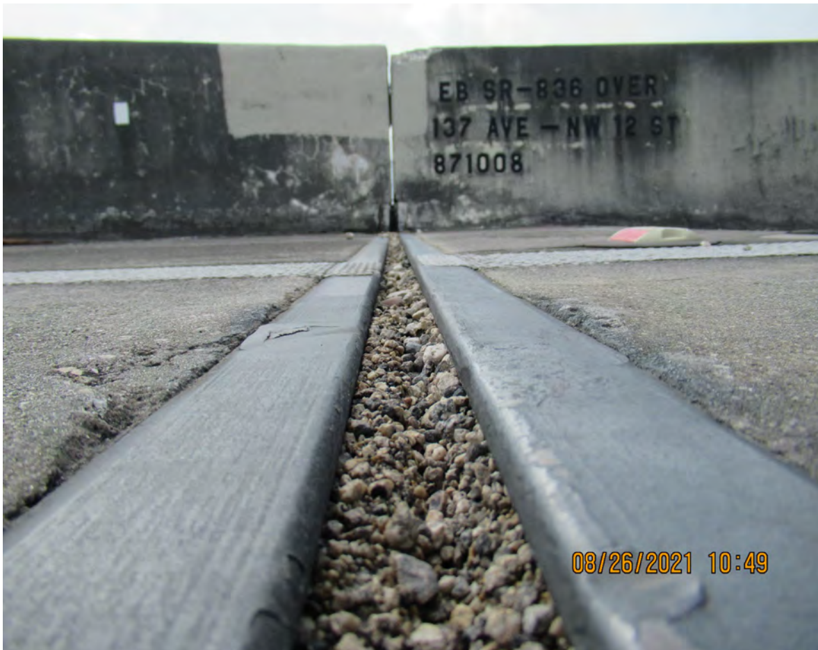
DEBRIS ON BRIDGE EXPANSION JOINT (BRIDGE No. 871008) (TYPICAL THROUGHOUT)
