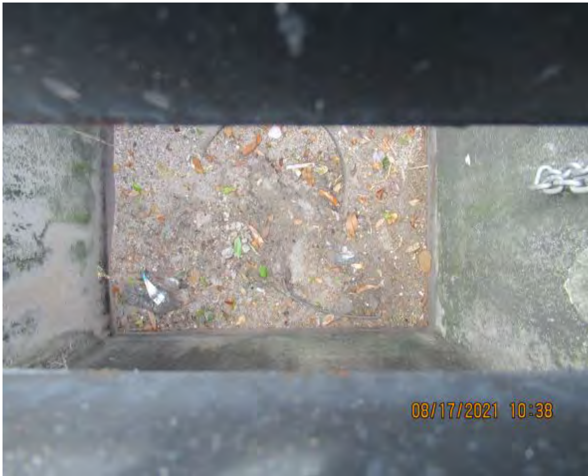
SILTED DRAINAGE STRUCTURE (TYPICAL THROUGHOUT THE CORRIDOR)
