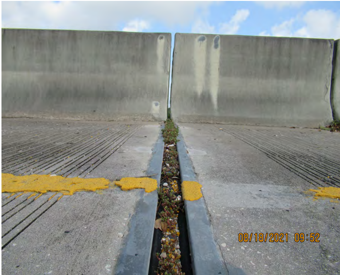
DEBRIS ON BRIDGE JOINT (BRIDGE # 871024)
