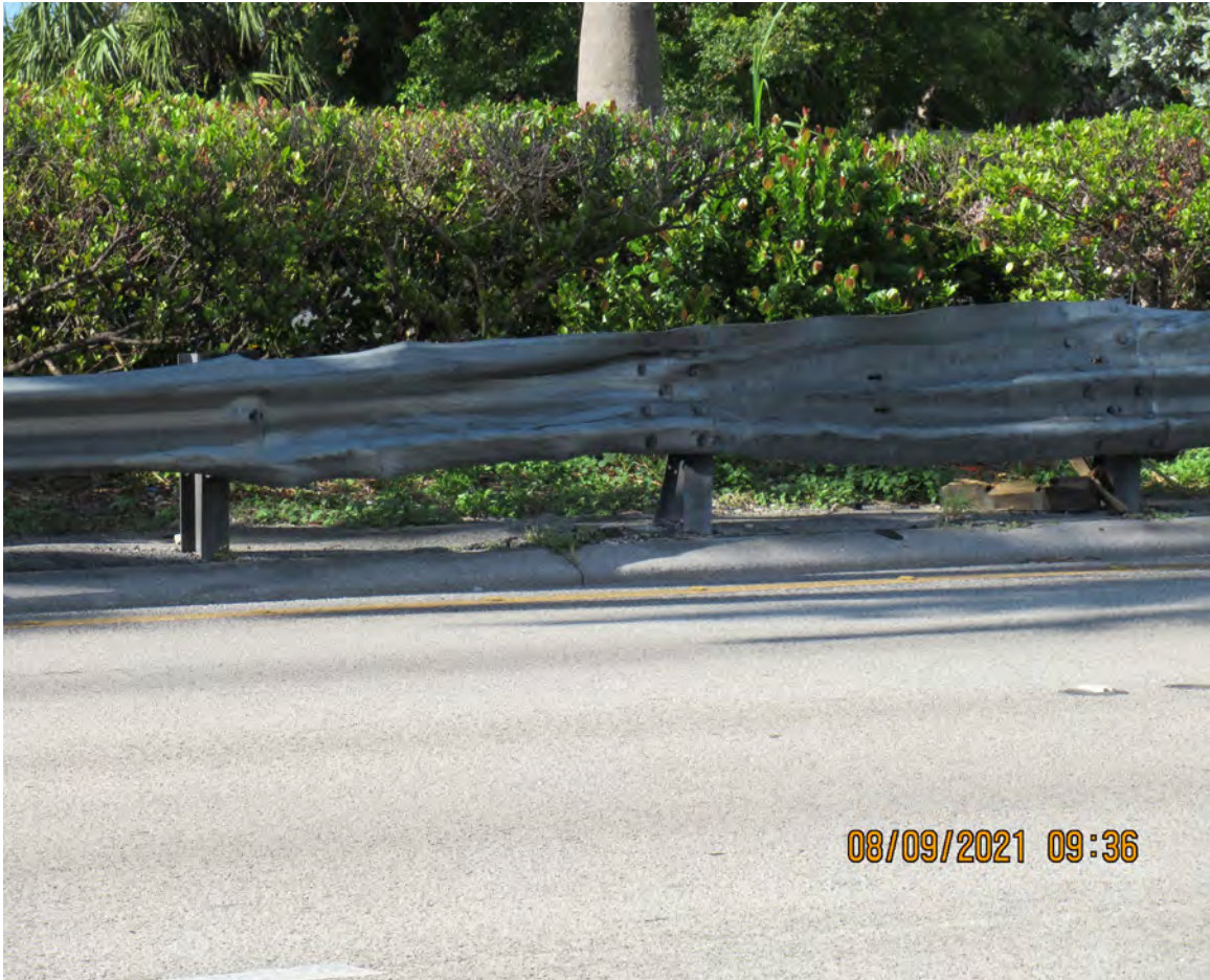
DAMAGED GUARDRAIL
