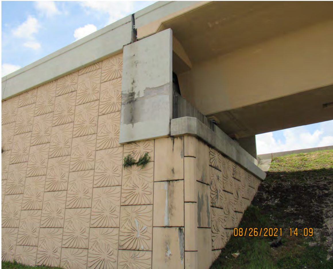
DETERIORATED CLASS V COATING AT BENT 12 (BRIDGE # 871050)
