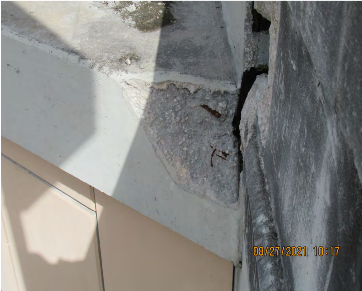
SPALL ON ABUTMENT 1 (BRIDGE # 870966)
