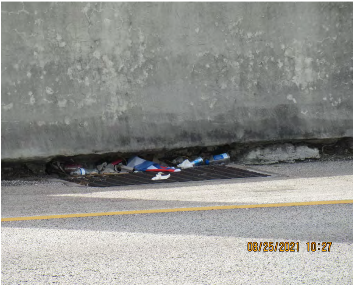
TRASH AND DEBRIS ON DRAINAGE STRUCTURE (TYPICAL AT VARIOUS LOCATIONS)
