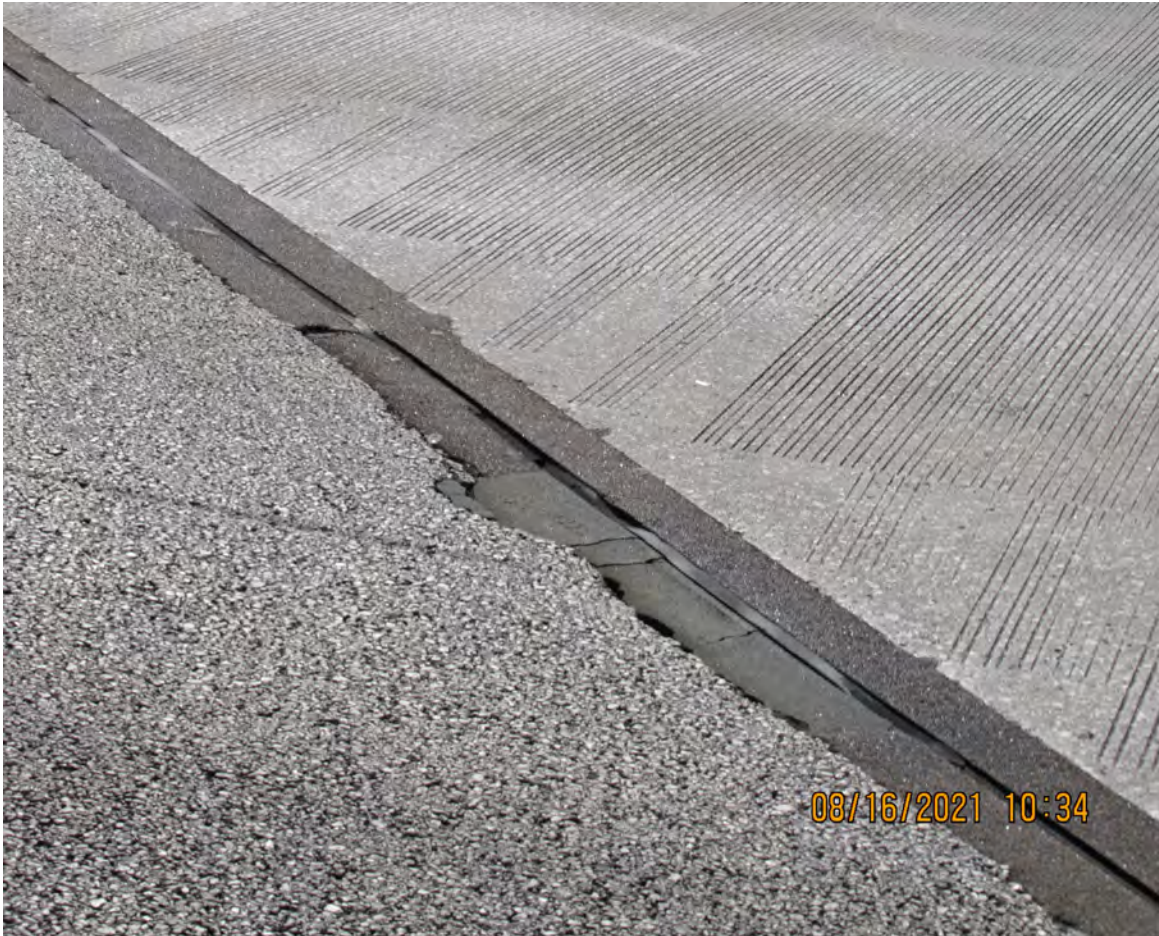
DETERIORATED POLYMER NOSING BRIDGE JOINT HEADER (BRIDGE # 870522)
