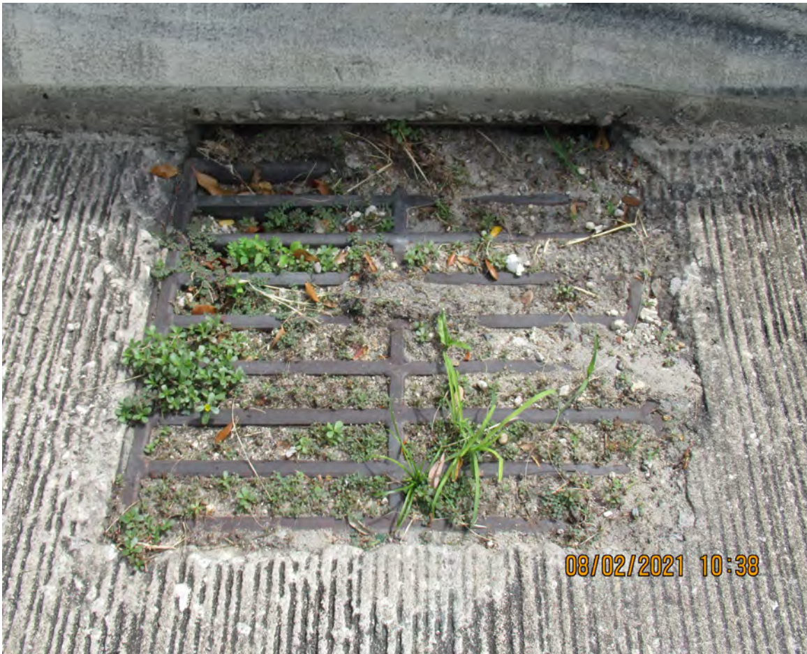
SILTED BRIDGE DRAINAGE INLET BRIDGE #870559 (TYPICAL AT VARIOUS LOCATIONS)
