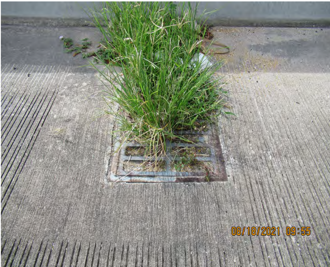
SILTED BRIDGE DRAINAGE (BRIDGE # 871024) (TYPICAL THROUGHOUT THE BRIDGE)
